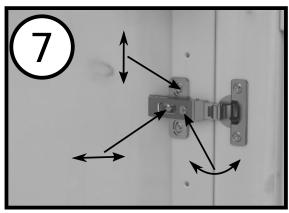
To adjust the position of the door use the adjusting screws.
